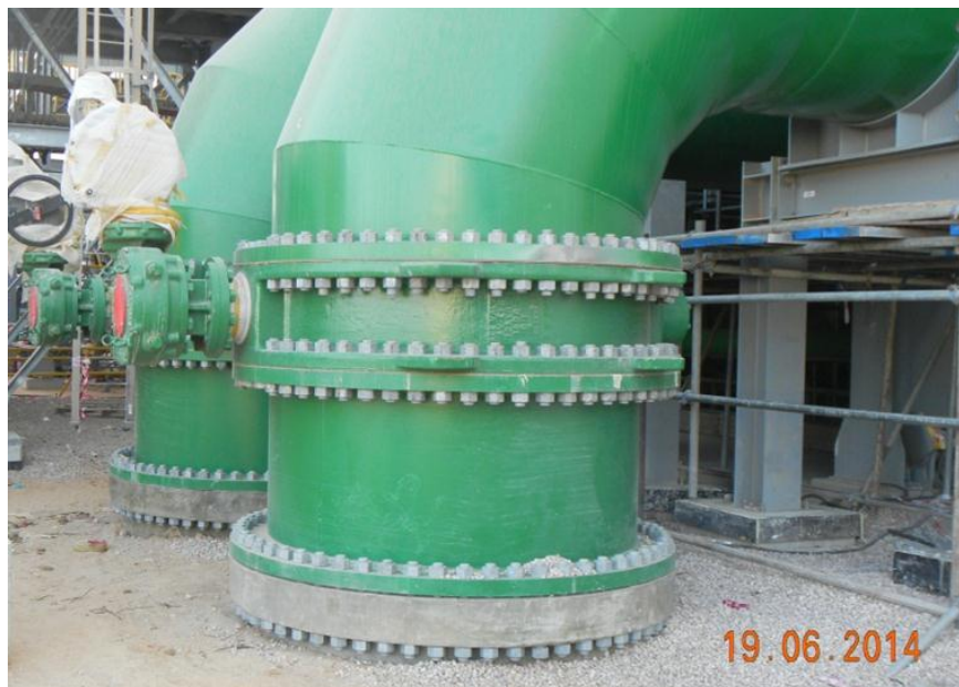
Photo 9. Flanged Connection of Return Lines GRP Headers to DN1800 Turbine Condensers
