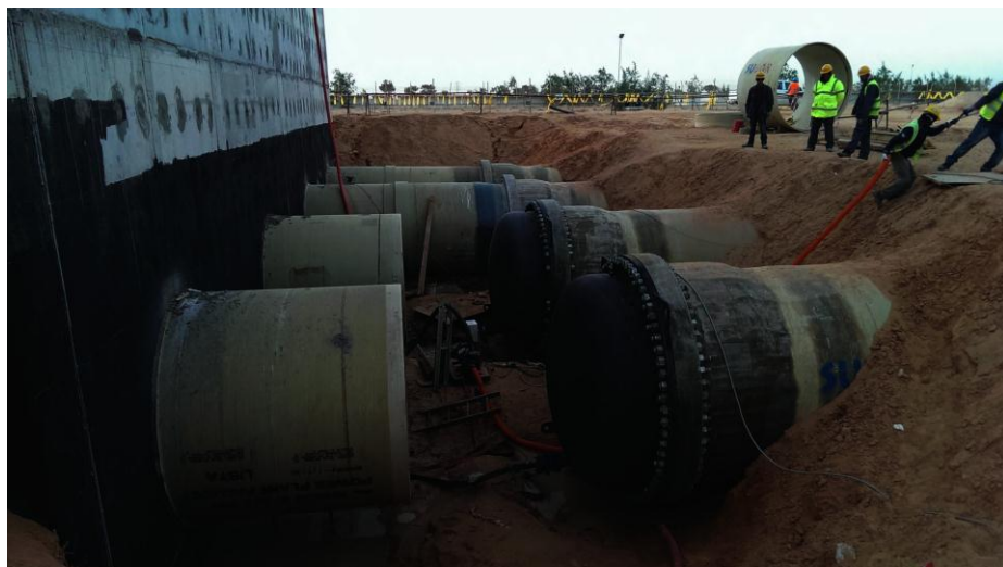
Photo 11. Hydrostatic Site Test of Unit 4 Cooling Water Return Line between Turbine and Surge Chamber with DN2500 Test Cover on Surge Chamber Side (January 2014)
