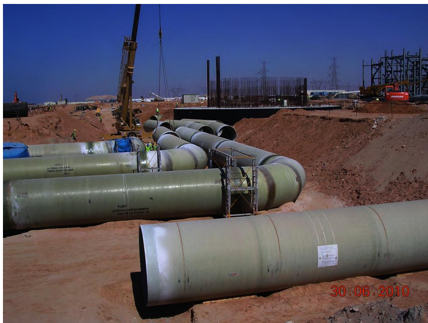
Photo 8. Installation of DN2500 GRP Cooling Water Pipes
