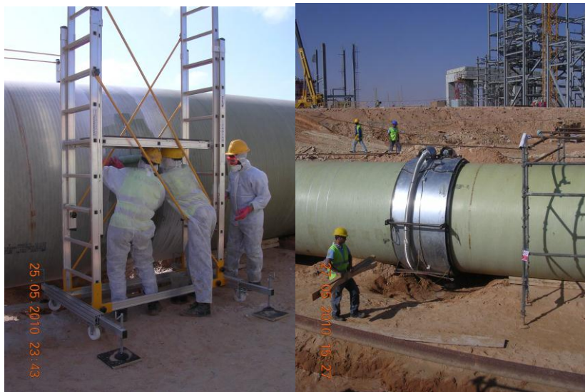
Photo 10. Butt and Wrap Connection of Pipe Pieces and Post Curing of these Connections
