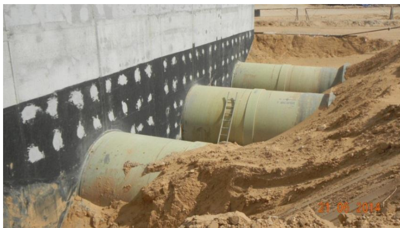
Photo 17. Connection of GRP Pipes to Surge Chamber with "Short Pipes" and REKA Couplings
