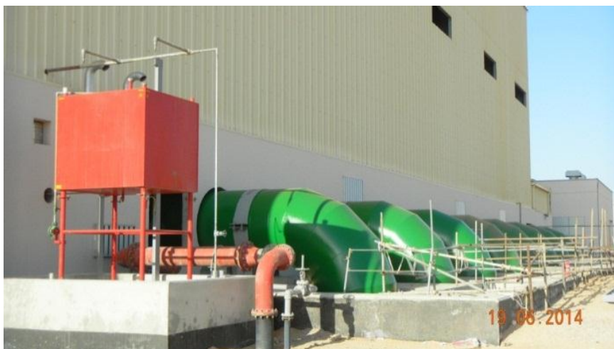
Photo 5. Connection of Eight DN1800 Supply Water Pipes from Intake Sea Water Pumps inside the Cooling Water Pump House to Intake Header
